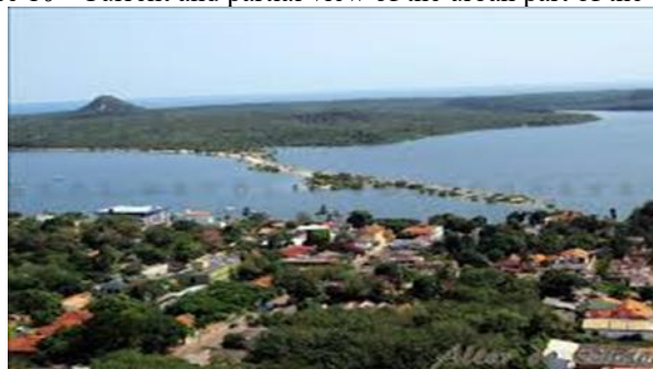
Figure 10 - Current and partial view of the urban part of the village
