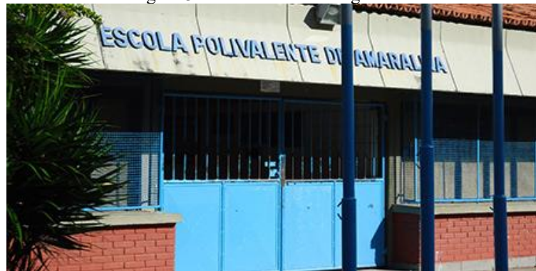
Figure 3. PSA school building facade.
