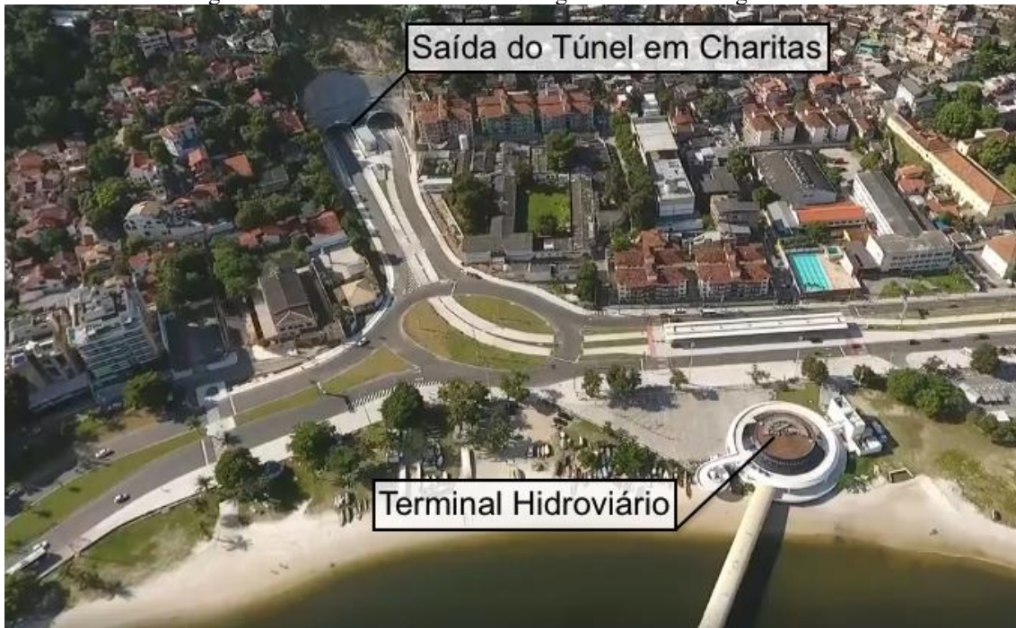
Figure 4: Entrance to the Tunnel through the Charitas neighborhood
