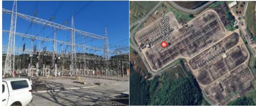
Figure 1 - Installation of SE A
