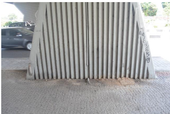
(e) Cracking and peeling of concrete in a column (SO 1)
